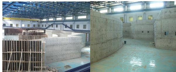
Figure 8: Current radiation shielding wall construction.
