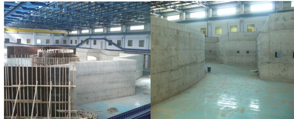
Figure 8: Current radiation shielding wall construction.
