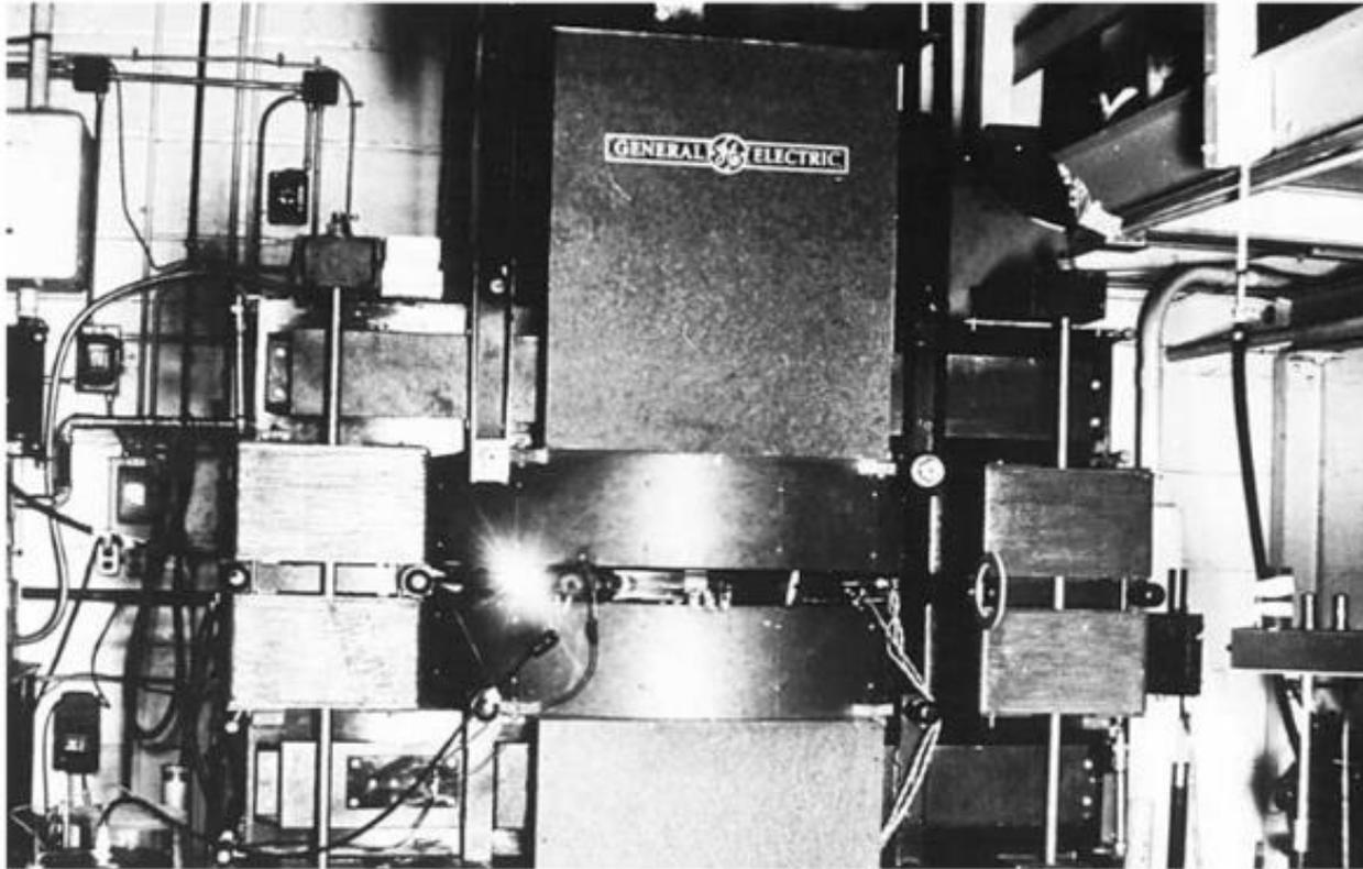
This 300 MeV electron synchrotron at the General Electric Co. at Schenectady, built in the late 1940s. The photograph shows a beam of synchrotron radiation emerging.
