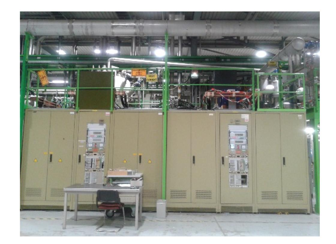
The selected powering topology is to connect two existing 15 kA power converters in parallel, to provide the 30 kA.
