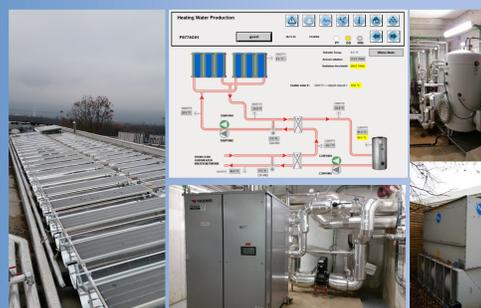
B774 Actual implementation of the solar collectors with its control panel interface
