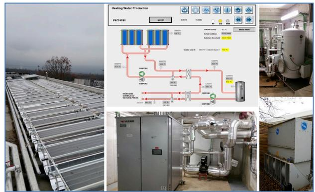
Figure 6: B774 Actual implementation of the solar collectors with its control panel interface.
