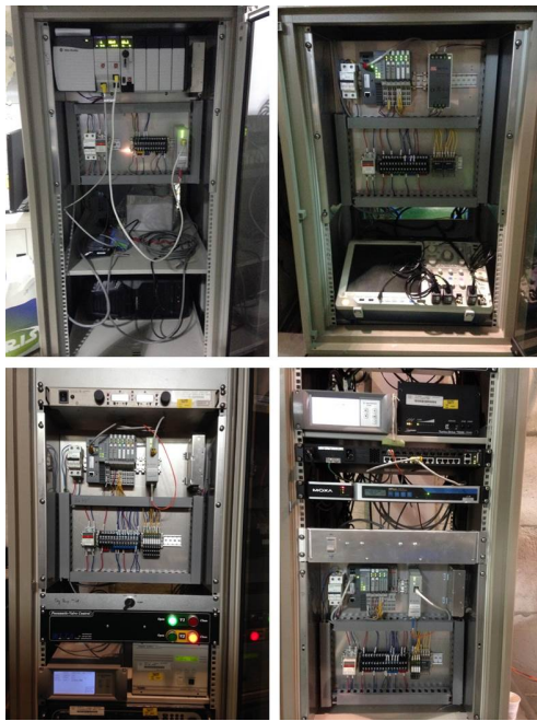
Figure 2: Installed chassis on each platform to configure the vacuum interlock system of the ECR ion source.
