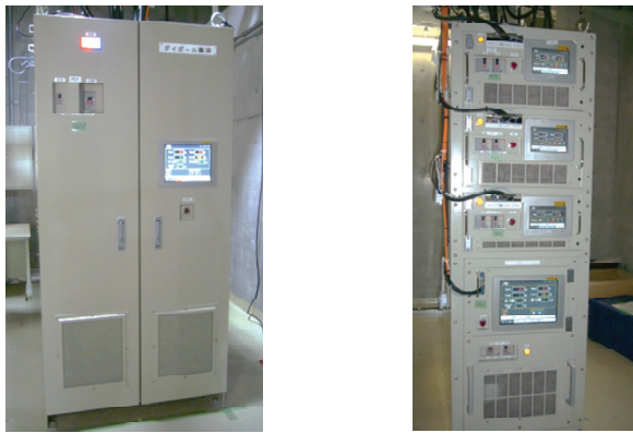
Figure 3: Pictures of the new power supplies for the normal-conducting magnets. The left photo shows a power supply for a dipole magnet and the right shows four steering magnet power supplies installed in a rack.
