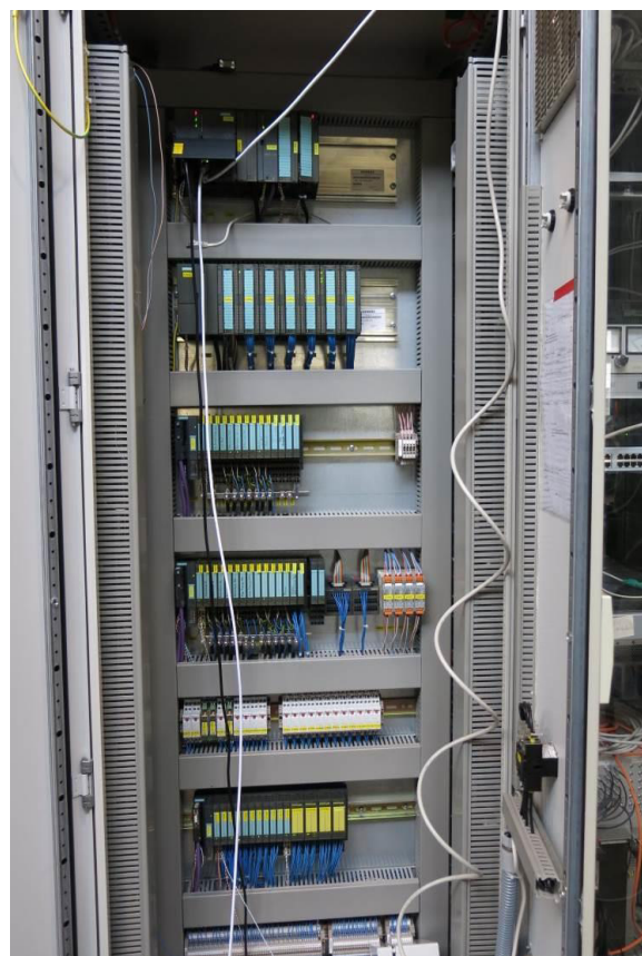
Figure 4: Main cabinet with PLC and 3 ET200S systems.
