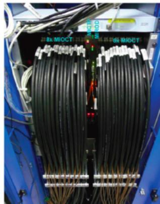
Figure 2: The final MuCTPi as it is installed in the ATLAS experiment.
