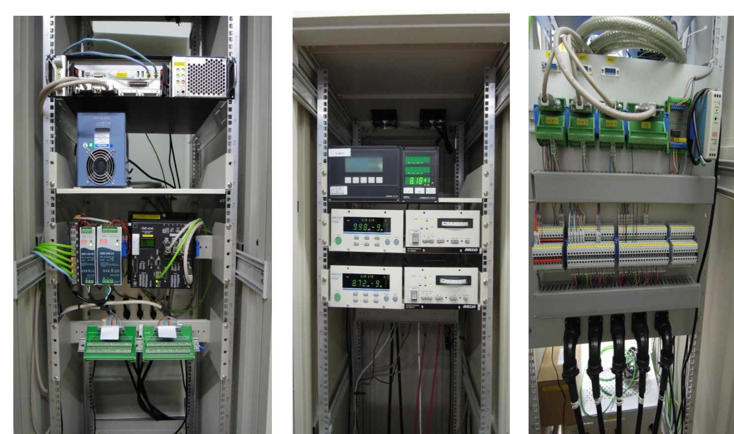
Control rack layout of IU22 for TPS.
