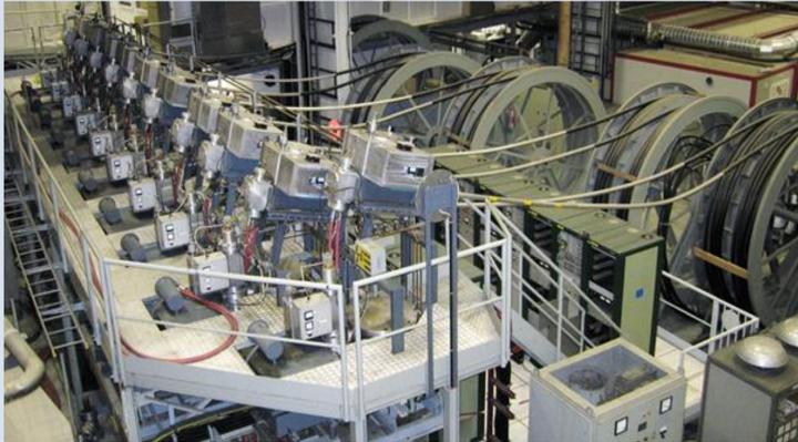
Antiproton Decelerator (AD) extraction kicker system layout
