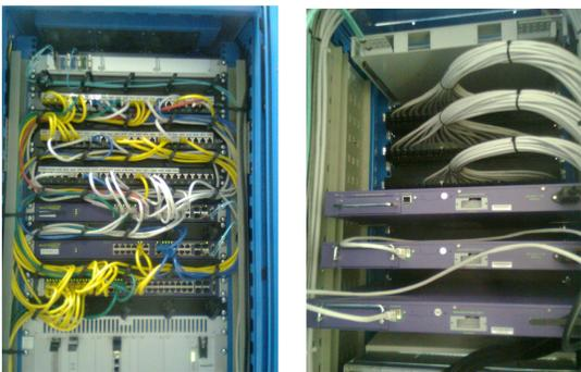
At the time of writing more than 110 peripheral switches, Summit X350 and X150 made by Extreme Networks, are installed in the 65 racks that host the control system and diagnostics devices, distributed along the FERMI buildings. A grand total of about 1800 devices are connected to the control system network.
