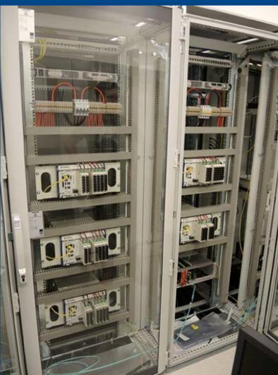
Full-scale system deployed at facility site in data center. Power converters are remotely controlled via optical fibers at distances from 25 to 120 meters.
