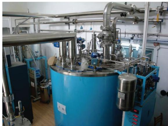
Figure 2: The large scale helium refrigerator on site.
