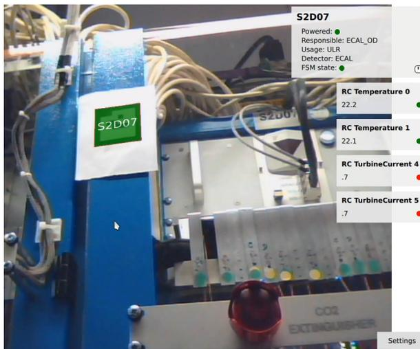
Figure 3: Augmented reality used in the CMS DCS to overlay controls system data on the operator's view as this walks around in the underground counting rooms (Courtesy of CMS DCS).
