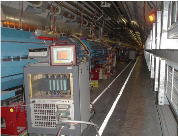
Figure 2: Bake-out mobile cabinet in the LHC Tunnel.
