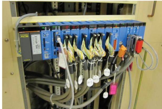
Figure 5: FA-M3-based IOC for vacuum control. From left to right, a Power Supply, a normal sequence CPU, an F3RP61 CPU and I/O modules.
