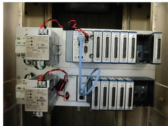
Figure 6: cRIO under installation. The light blue cable is for EtherCAT that connects main unit (upper) and extension unit (lower).
