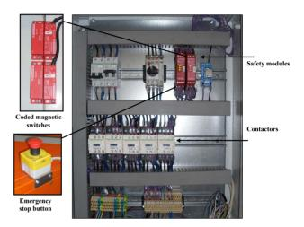
Figure 3: The LASER safety control system.
