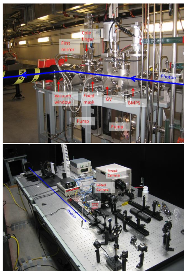
Figure 1: (top) Installed visible synchrotron light monitor (SLM) beamline components inside the NSLS2 storage ring tunnel; (bottom) Optical table setup in the SLM hutch.
