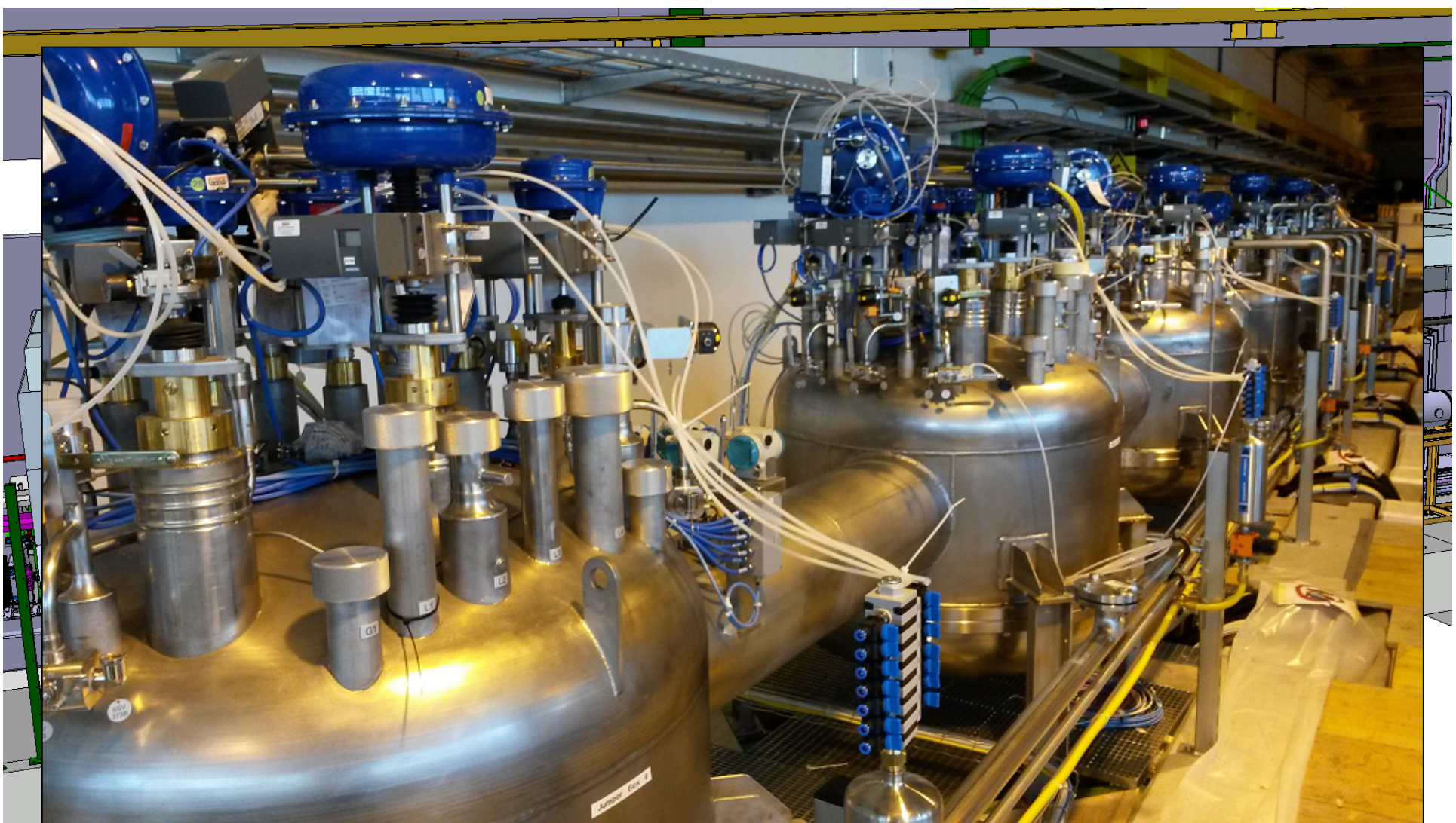
Cryo Cold Line & Jumper Boxes instrumentation: installation finished Pressure tests done on Cold Line.
