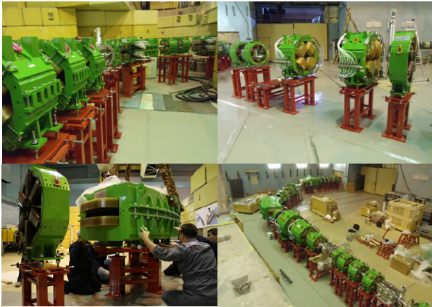
Figure 4: UL Primary beamline, UR 2 quads, 2 6-poles and 1 8-pole in secondary beamline, LL Installation of D1 secondary dipole on its stand, LR End of primary and secondary beamlines with vacuum elements assembled.
