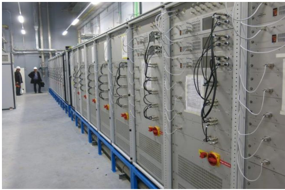
Figure 6: Solid state 88.0525 MHz amplifiers.
