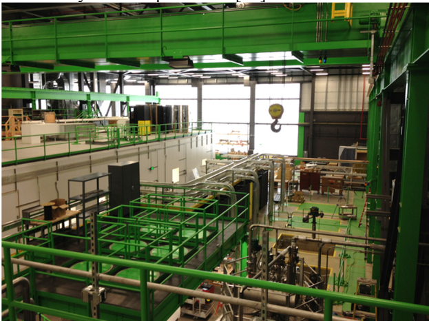
Figure 6: Newly constructed SRF Highbay at MSU.
