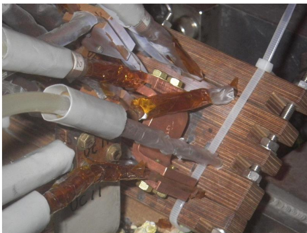
Figure 7: Normal connection between two hollow-conductors with electrodes (left), and damaged electrodes (right).
