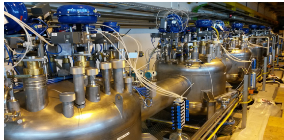
Figure 1: Cryogenic distribution line feeding the SC linac with liquid He at 4.5K.
