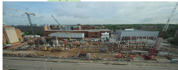
Figure 1: Layout of the FRIB driver accelerator, target and fragment separator (colored areas) and existing infrastructure (top); photograph showing FRIB civil construction (bottom).
