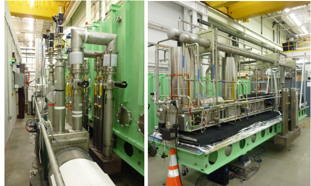
Figure 2: Left: test bunker with cryogenic distribution via U-tube connections. Right: prototype \beta_0=0.085 cryomodule housing 2 cavities and a solenoid.
