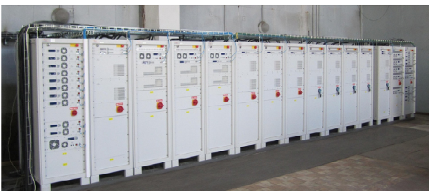
Figure 6: The power supply cabinets.
