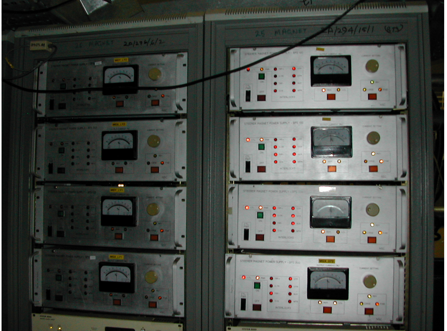
Power supplies for beam transport systems
