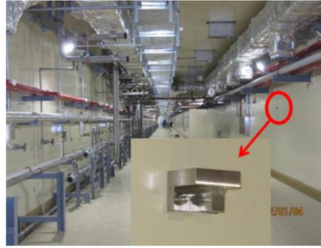
Figure 5: The target holder for alignment network in the accelerator tunnel.
