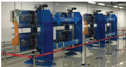
Figure 6: Two undulators installed at the hard X-ray undulator hall. They are 1st undulator line and facing the wall.
