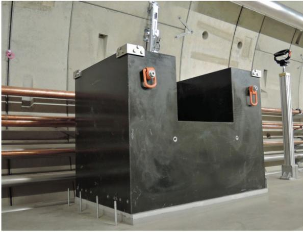
Figure 11: Support granite for the mirror chamber, installed on top of a concrete base.
