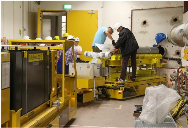
Figure 3: Test installation of the injector dump [11]. The dump is placed on the exchange device ready to be moved into its concrete housing to the right.
