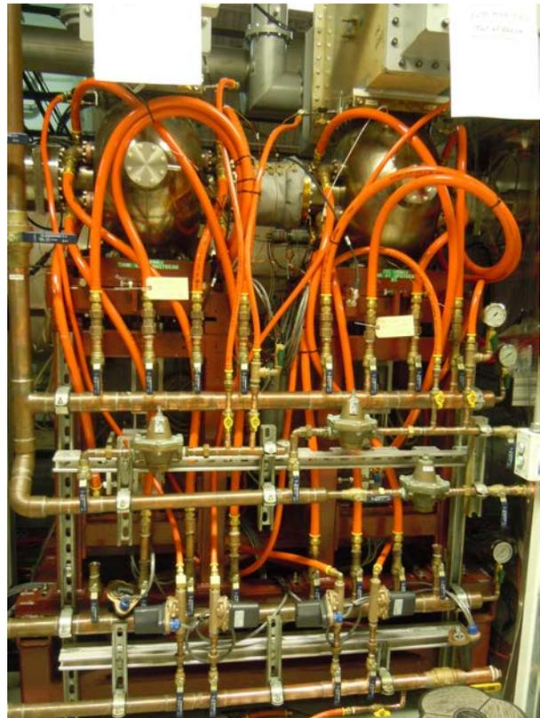
Figure 4: 500 MHz cavities with water manifold installed in the RHIC tunnel. The RF power is fed from the two waveguides on the top of the cavities.
