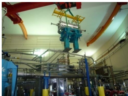
Undulator installation
