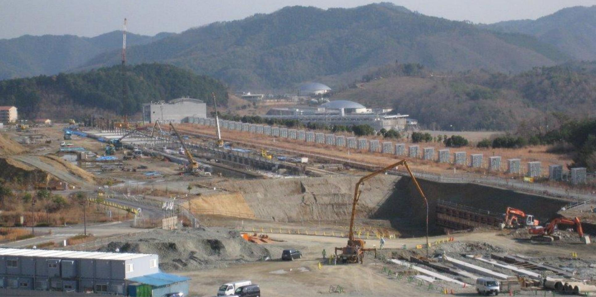
Excavating 17 m deep at undulator area, replaced with crashed stones on base rock, which took 8 month. Only -1.7 mm vertical movement was observed for 2 year after completion. Extremely stable basement was made for undulator hall.
