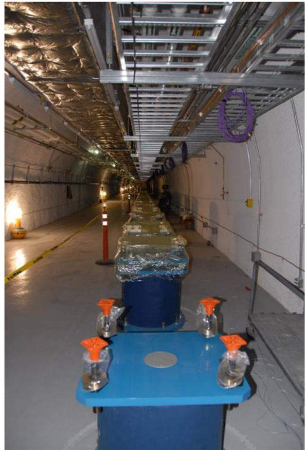
Figure 14: Initial installation of the fixed support systems for the LCLS undulators.
