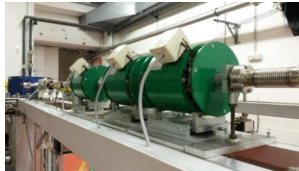
Figure 2: Three skew quadrupole magnets in the first recirculation of the S-DALINAC. They will be relocated in the second loop in the described SFSDS lattice above.
