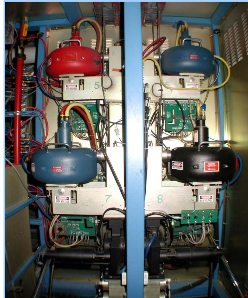
Inside a transmitter: 8 klystron (4 to be seen) powered by one power supply
