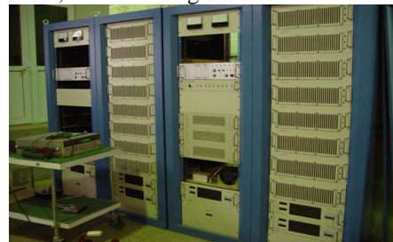
Fig. 4 The 6kW driving power amplifier and monitoring devices
