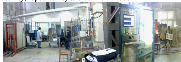
Fig.5 Acceptance of RF power generators and transmission lines
