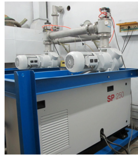
Figure 3: The new rough pumping stations of SSC and SFC
