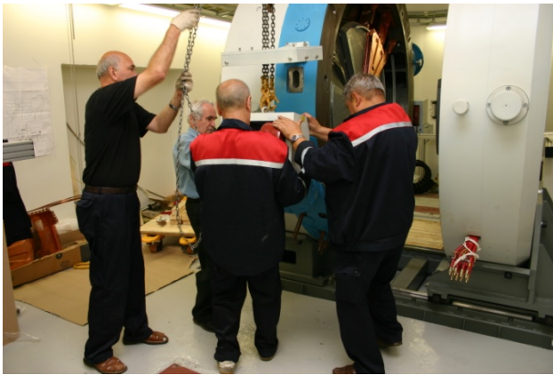
Figure 2: The NIEFA team installing the matching dipole. The cyclotron magnet opens sideways on precision rails.
