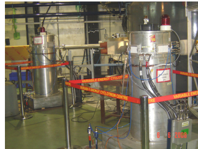
Fig.1. High power rf amplifiers installed at SCC Vault
