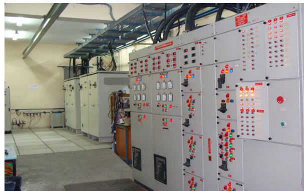
Figure 6: Anode Transformers & Local Control Panel showing monitoring, fault indications & controls.
