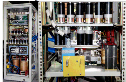
Fig. 12 Photos of main magnet power supply.
