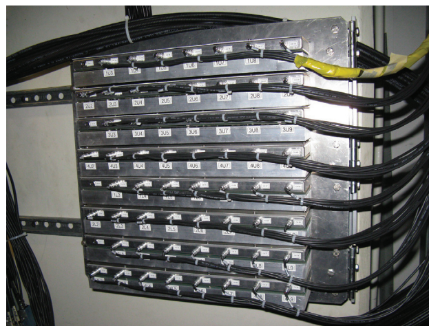
Figure 1: Cyclotron voltage probe detectors.
