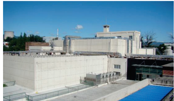
Figure 2: Main building of BRIF.
