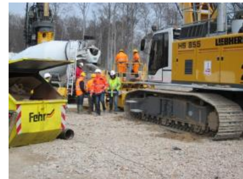
drilling of holes for pillars
