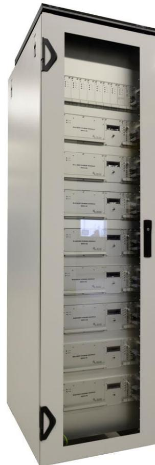
Figure 4: Magnet power supply cabinet.
