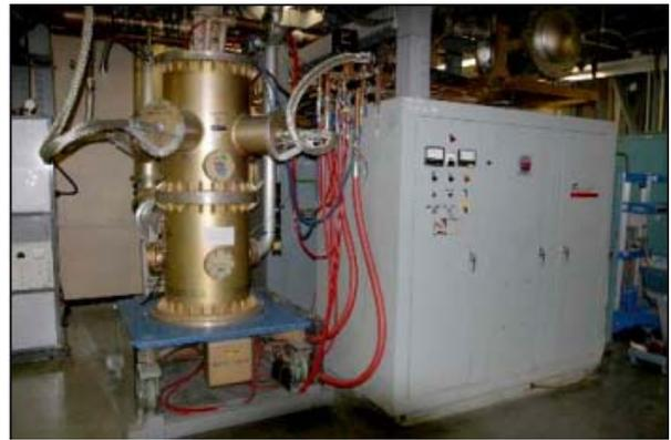
Figure 1: 201 MHz cavity amplifier and filament supply for the Burler 7835 triode.
