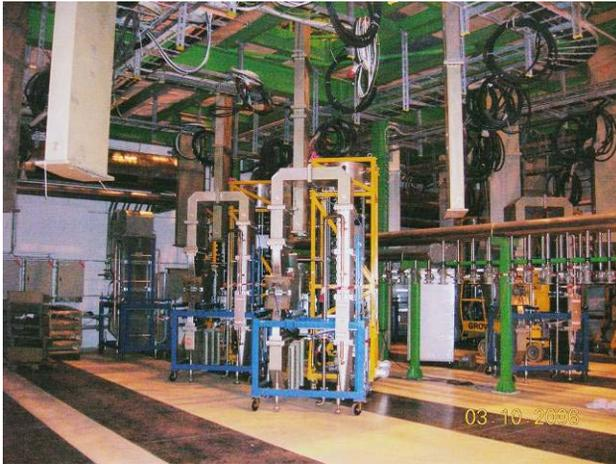
Figure 10: LHC klystrons.
