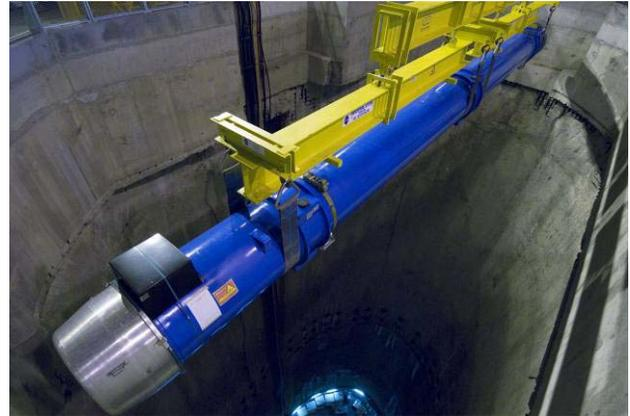
Figure 4: Lowering of the last dipole.
