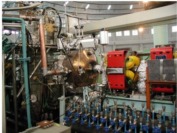
Figure 6: The HLS RF cavity installed on 800MeV electron storage ring.
