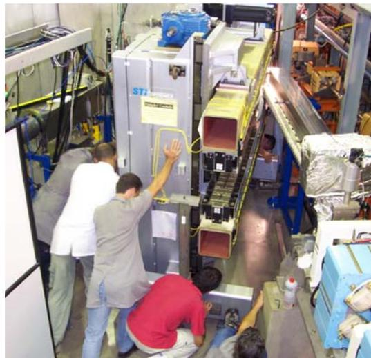
Figure 3: Bringing the 2.0 T wiggler into position.
