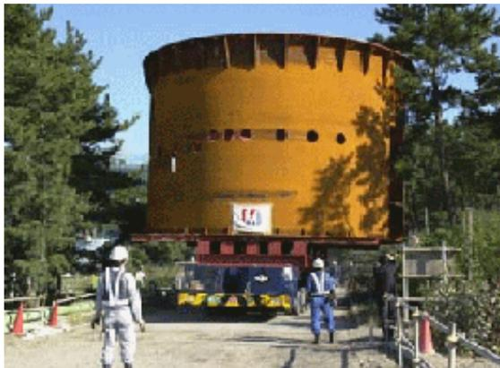
Figure 8: Transportation of the large outer liner along the road to the site of the MLF.
