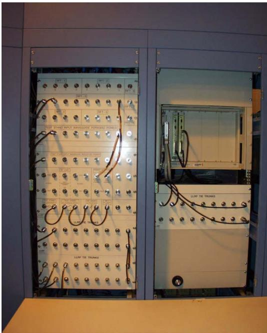
Figure 3: Low-level rf patchbay.
