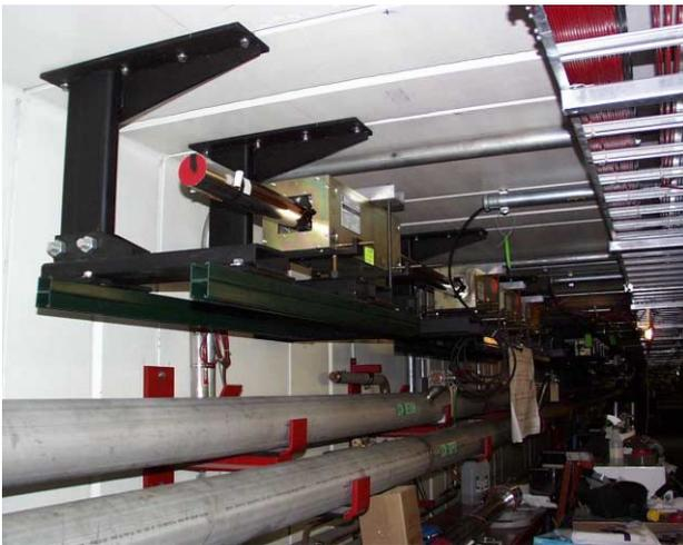
Figure 5: A section of the Recycler MI-30 straight section with the new cooling insert
