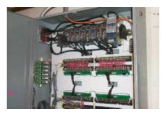
Figure 3: PLC in interlock chassis.
