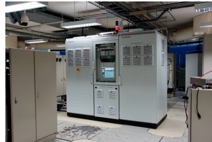
Figure 6: The new 80 kW solid-state RF amplifier.
