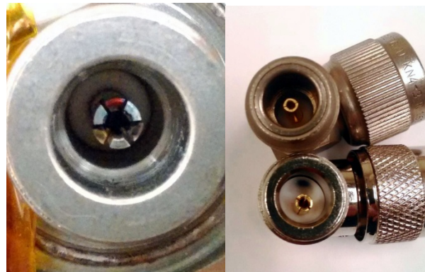
Figure 2: Burned feedthrough connector (left), damaged coaxial adapter connected to the feedthrough (right).
