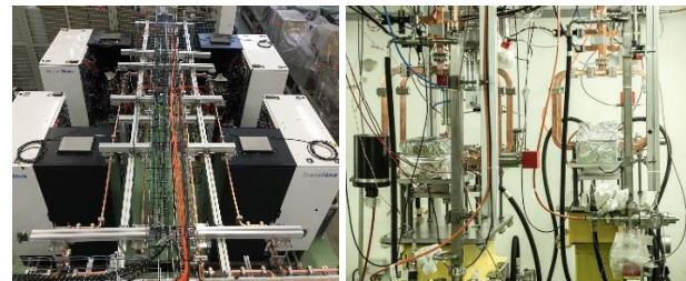
Figure 4: The modulators of Xbox-3 (left) and test slots C and D with structures installed (right).
