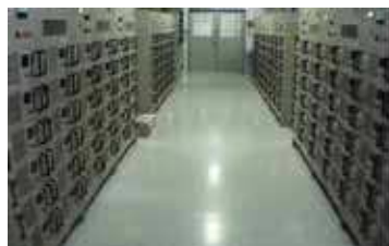
Fig.1-a. Steering magnet power supplies.
