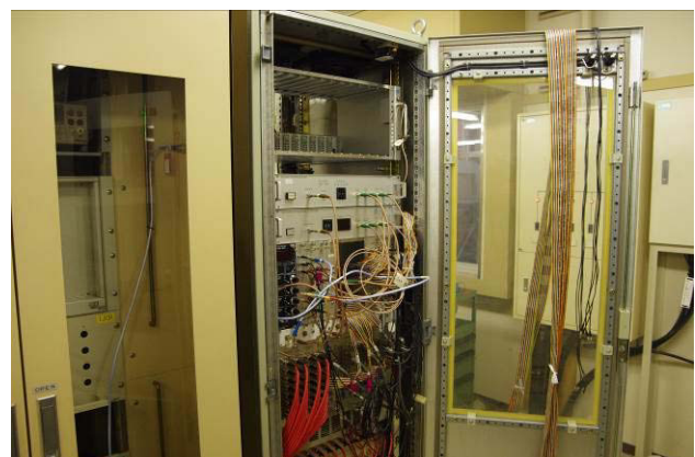
Figure 6: Loss monitor station at KEKB-D7 under installation work.
