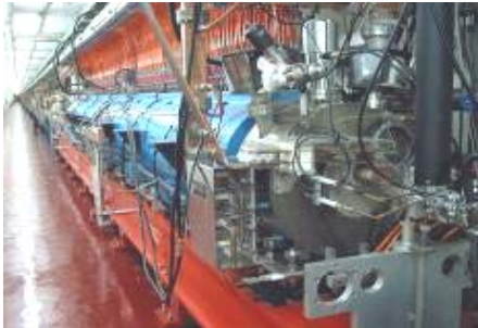
Figure 3: The BEPCII injector linac.
