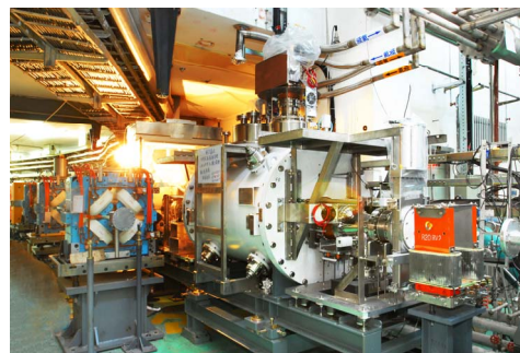
Figure 4: A superconducting cavity in installation.
