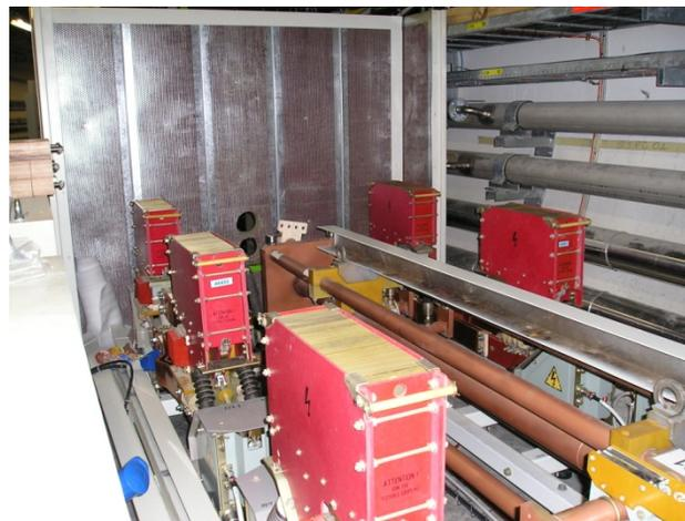
Figure 1: A view on the 13 kA switch unit for the dipoles.
